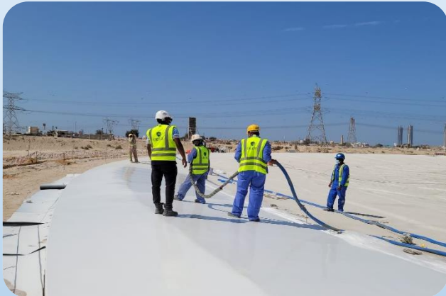
Belvin @ Meydan phase III application of DELTAShield Aqualine AL
